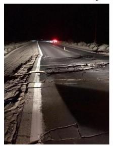
California State Route 178 SW of Trona, following the M7.1 earthquake. Road is now closed for repairs. USGS Photo
