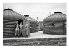
Last Week: Buckminster Fuller's Dymaxion Deployment Unit. Fuller began his "Dymaxion investigations in 1927, with a proposal for a mass-produced bathroom and a house. His early investigations coupled with the happy (if anecdotal) accident of seeing a grain bin, led him to develop the version of the Dymaxion Deployment Unit seen here. Commissioned by the US army for field housing, hundreds of these units were shipped to the Persian Gulf during World War Two.
