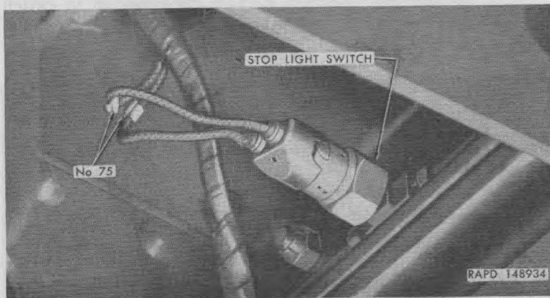
Figure 94. Stop light switch installed.
