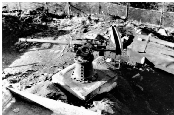
7A – 6 Pounder, 8 hundredweight Hotchkiss Gun. This gun was the standard examination service enforcer in the Coast Artillery Forts. It could fire 25 rounds per minute with a muzzle velocity of 1,818 feet per second (554 m/s) and an effective firing range of 4,000 yards (3,700 m).
