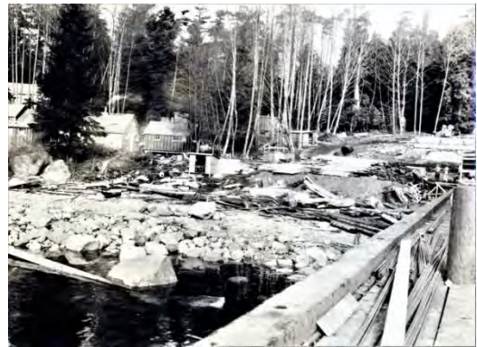
2B – Dock Construction. This photo provides a view of the dock area circa 1938/39. The dock boards have yet to be installed and it appears that the ground is being prepared for the Officers’ Quarters. The existing buildings appear to be short term construction sheds. 15FdMuseum989.154.56
