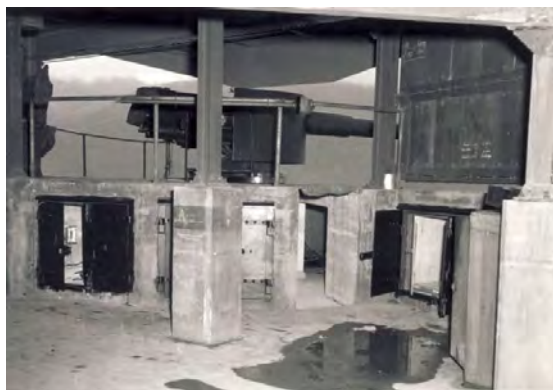
6H - 6-Inch Breech Loading Mark VII Gun. Interior view of #2 gun shows additional detail on the ammunition storage recesses and the support structure for the plastic armour system. 15FdMuseumRE.84.1081
