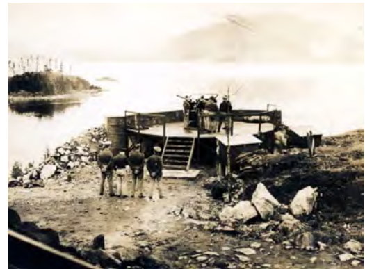
5D - 4.7-Inch Quick Firing Mark IV "B" Gun. This photo appears to show the #2 gun. There are no covers visible under the platform. The gun is covered with a gun tarp due to the inclement weather.
