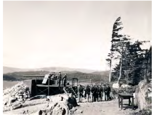
5B - 4.7-Inch Quick Firing Mark IV "B" Gun. This photo shows the #2 gun with 2 projectiles and a casing ready. The #1 gun is hidden under a camouflage net. 15FdMuseum985.88.185, 984.73.9n, 994.25.12
