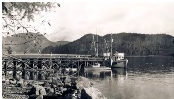
2E – Completed Dock. The view looking south towards Hardwicke Island. 15FdMuseum985.88.133
